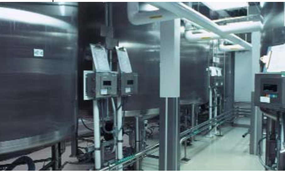
Photo Courtesy of Lockheed Greene Engineers, Inc.
